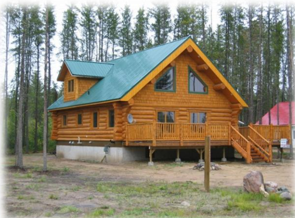
Figure 4: Cabins shown with metal and asphalt protected roofs, gravel/crushed rock material up to foundation and fuels removed and/or thinned within home protection zone and outward. No fuels stacked within 10 m of structure. Negative observation is non-enclosed stilt deck on log home constructed of combustible material. Homeowner can either sheath or screen under deck similar to picture on right, or rake any fine fuel accumulations as required to remove the hazard.
