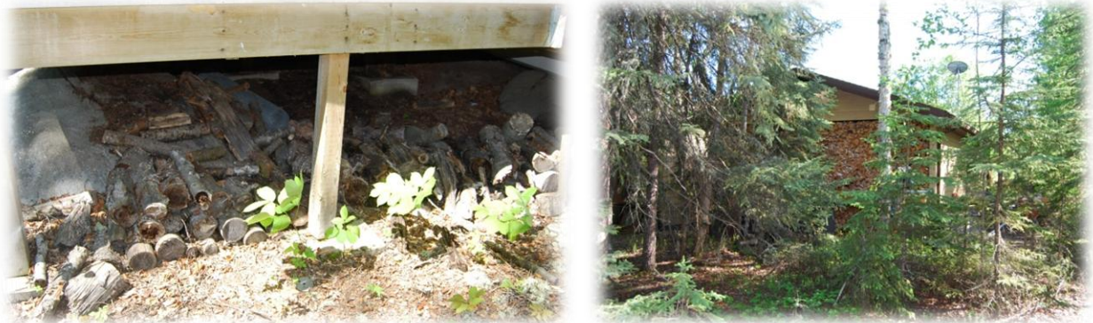
Figure 2: Firewood stacked too close to structures provides ignition points and fuel during wildfires (ember accumulators)
