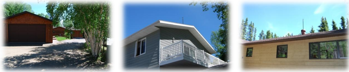
Figure 6: (Left) Well-maintained yard with spruce & surface fuels removed from home ignition zone. (Center and Right) Permanent sprinklers attached to homes complimenting FireSmart principles within the properties.
