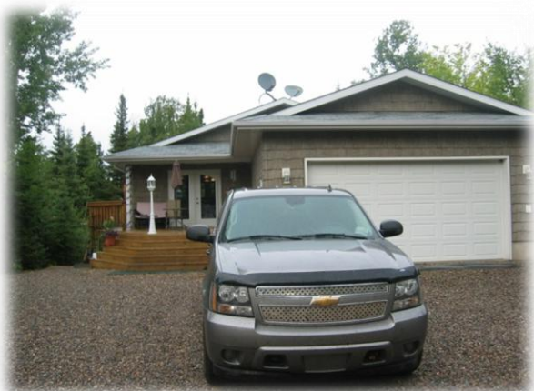
Figure 4: Cabins shown with metal and asphalt protected roofs, gravel/crushed rock material up to foundation and fuels removed and/or thinned within home protection zone and outward. No fuels stacked within 10 m of structure. Negative observation is non-enclosed stilt deck on log home constructed of combustible material. Homeowner can either sheath or screen under deck similar to picture on right, or rake any fine fuel accumulations as required to remove the hazard.
