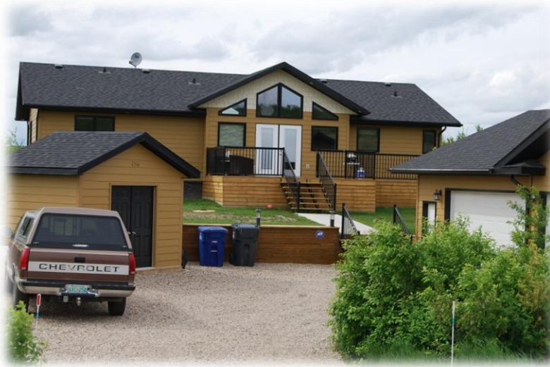
Figure 5: FireSmart home with enclosed deck, maintained lawn up to the structure and only deciduous shrubs nearby.
